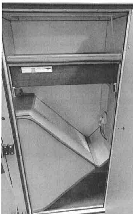
Fig. 6 Exhaust air filter and exchanger
