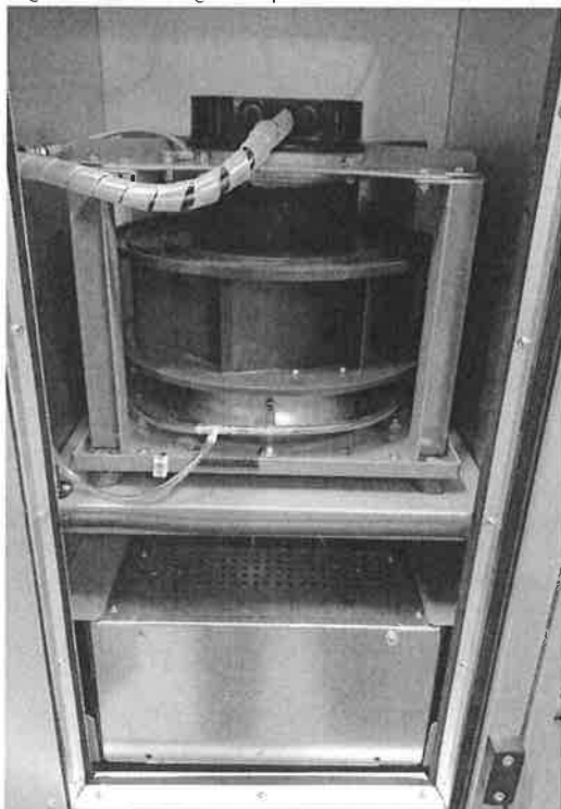
Fig. 5 Supply fan with electric heater
